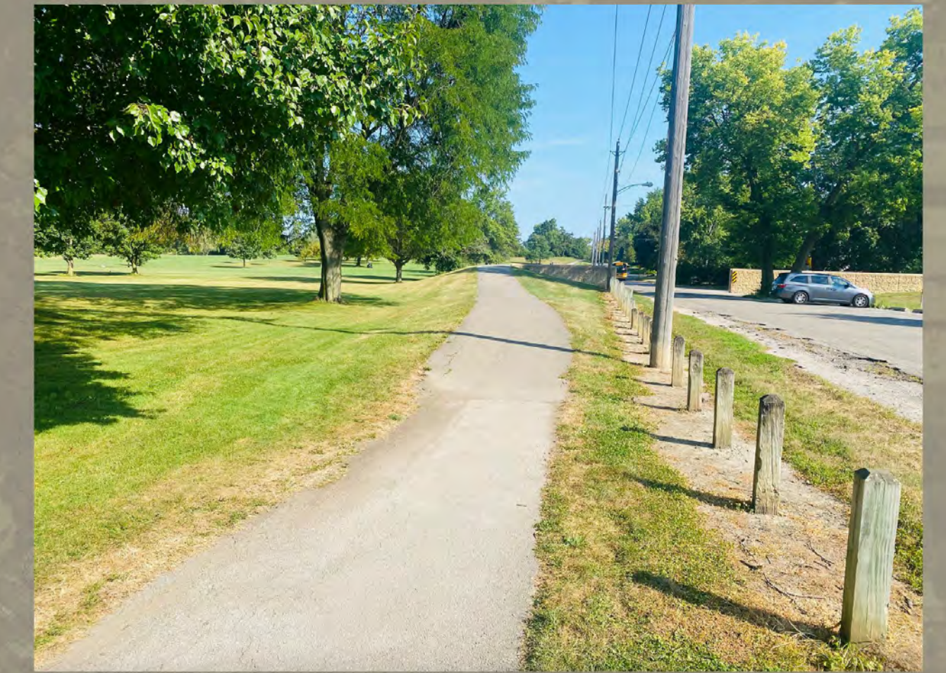
EXISTING HARTMAN ROAD TRAIL. MASTER PLAN SPECIFIES INCREASING TO 12' WIDTH
