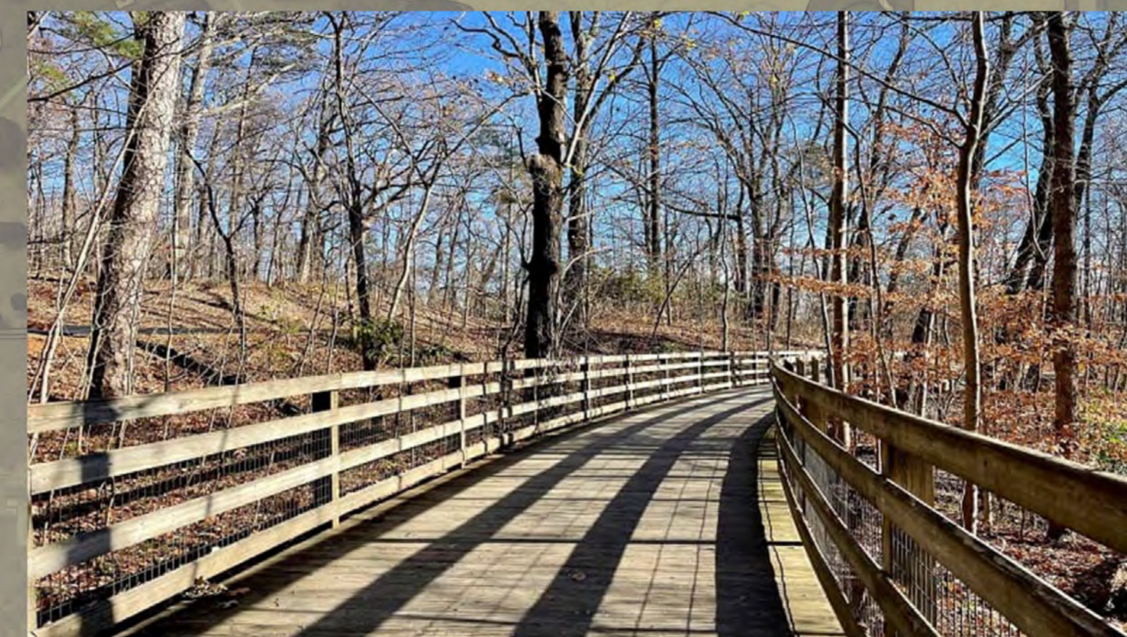
EXAMPLE OF BOARDWALK TRAIL TRAVERSING OVER NATURAL LANDSCAPE OR FLOOD-PRONE AREA ALONG THE ST. MARYS RIVER
