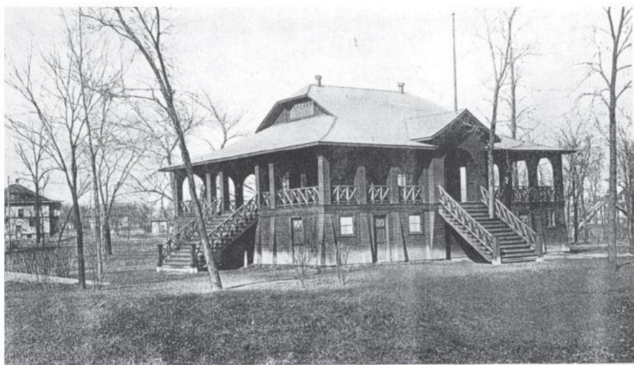
Figure I.10 The newly constructed refectory/bathhouse/comfort station located on the central island in the Lagoons, 1916. 1916 Annual Report, p. 34. Courtesy of Fort Wayne Parks & Recreation.
