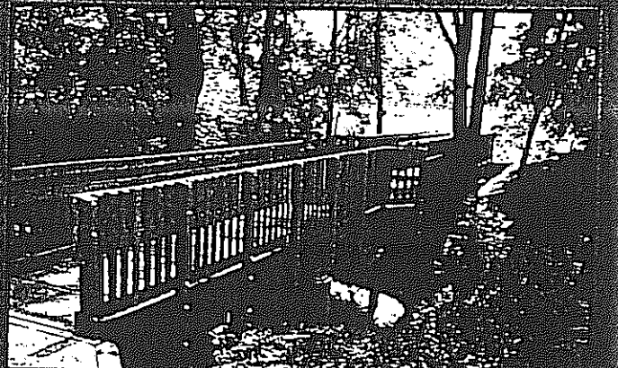
This is one of four FiRP® bridges at the Browns Ferry Park in Tualatin, Oregon. Note the 2 x 4 balusters and observation area.
