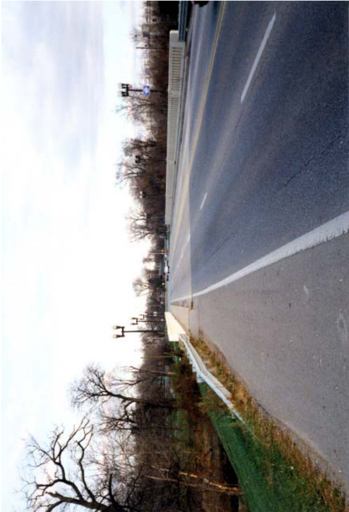
Figure III.1 Jefferson Boulevard bridge, with the narrow sidewalk being the only pedestrian connection between East Swinney Park and West Swinney Park. LANDSCAPES L.A. • Planning • HP.
