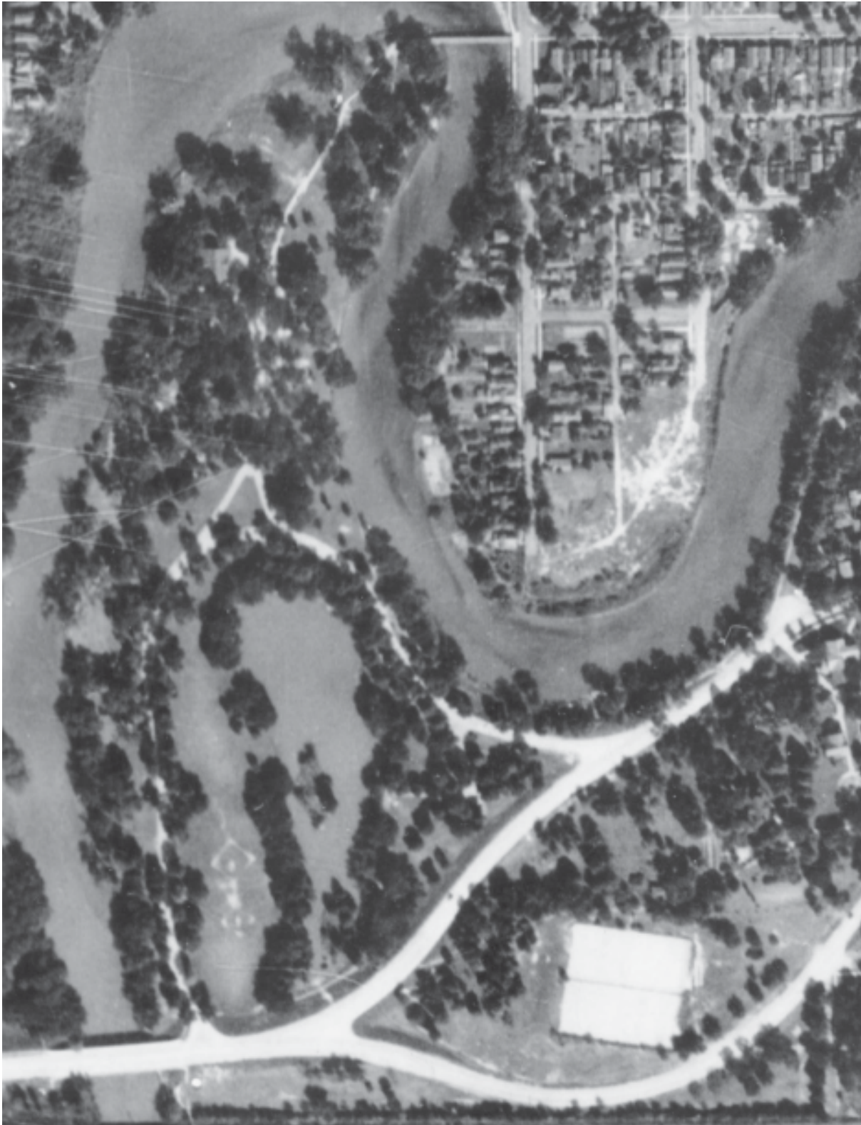
Figure I.11 Aerial photograph of East Swinney Park, 1938. The realignment of park drives to accommodate the extension of Washington and Jefferson Boulevards had recently been completed. Courtesy of Indiana State Archives.
