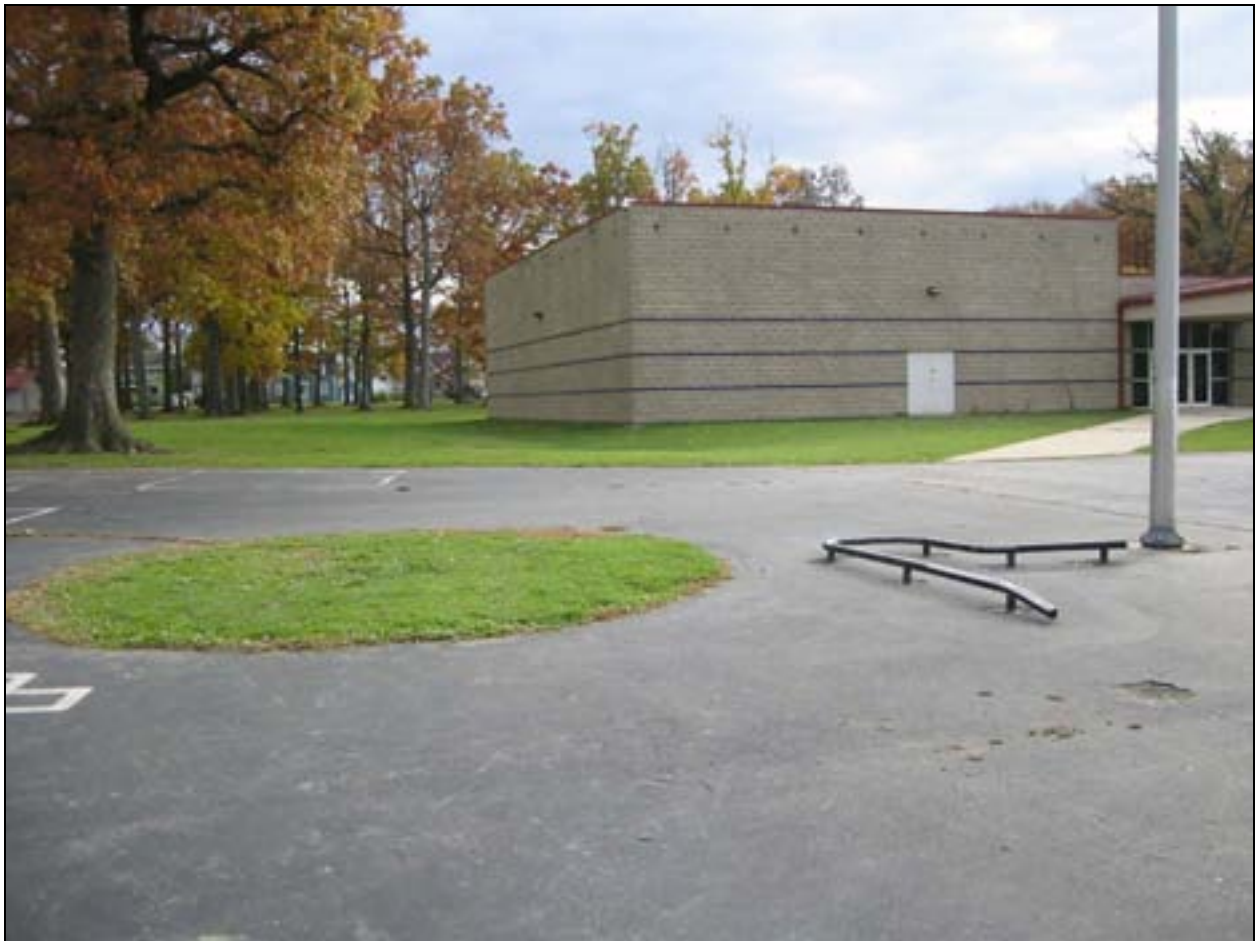
Figure IV.18 The Weisser Park Youth Center is used by children and residents of all ages, while the adjacent asphalt play area visible in the foreground is primarily used by the nearby Weisser Park School. Features of the play area include a low, metal rail, likely used for skateboarding. (R-FWP-WEI-CT- (10).jpg) Courtesy Heritage Landscapes.
