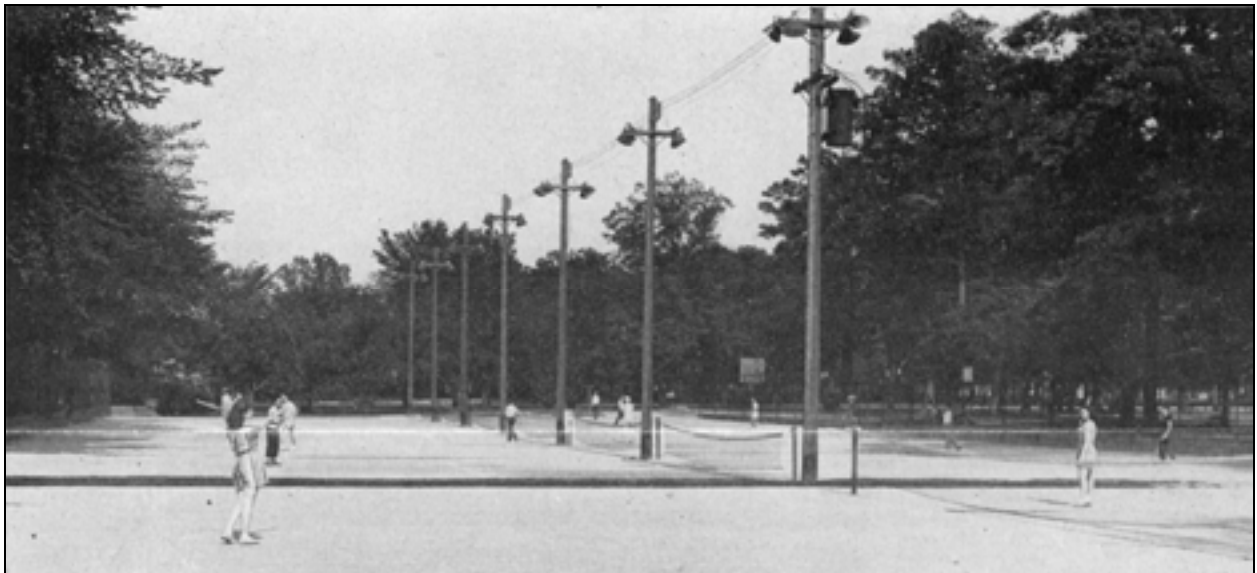
Figure II.12 Several tennis courts were constructed at Weisser Park. The courts became extremely popular and in circa 1939 floodlights were installed, seen here down the centerline of the image. The installation of the lights allowed the courts to be used into the evening hours. (R-FWP-WEI-Mun-Rev-07-08-Tennis-1941-pg4.jpg) Courtesy Fort Wayne Parks and Recreation.
