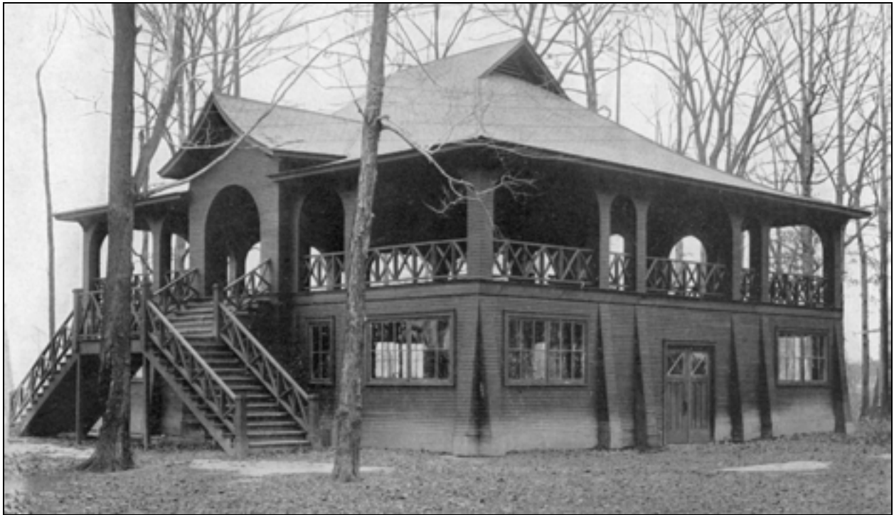
Figure II.7 The rustic style, wood-frame two-story pavilion, shown here shortly after completion in 1917, was set among the oak and hickory trees, creating a large social gathering space within the park. (R-FWP-WEI-Brd-Ann-Rpt-Pavilion-1917.jpg) Courtesy Fort Wayne Parks and Recreation.
