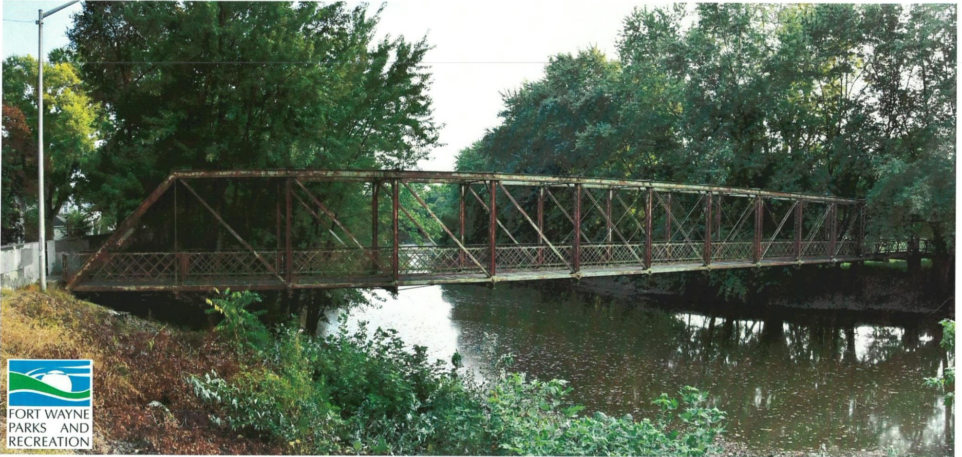
Mechanic Street Bridge
