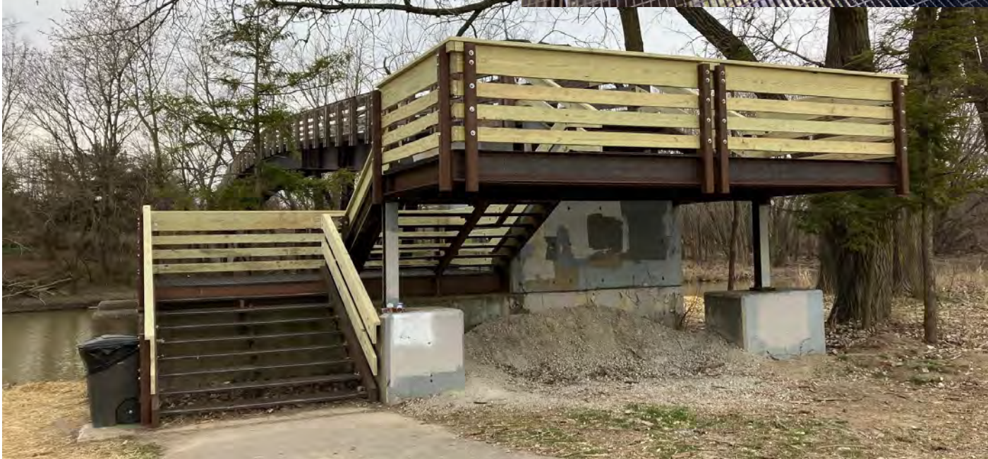
Old Fort Bridge
