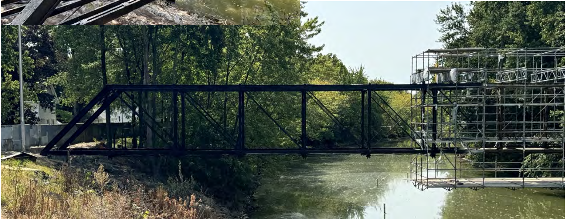
Mechanic Street Bridge
