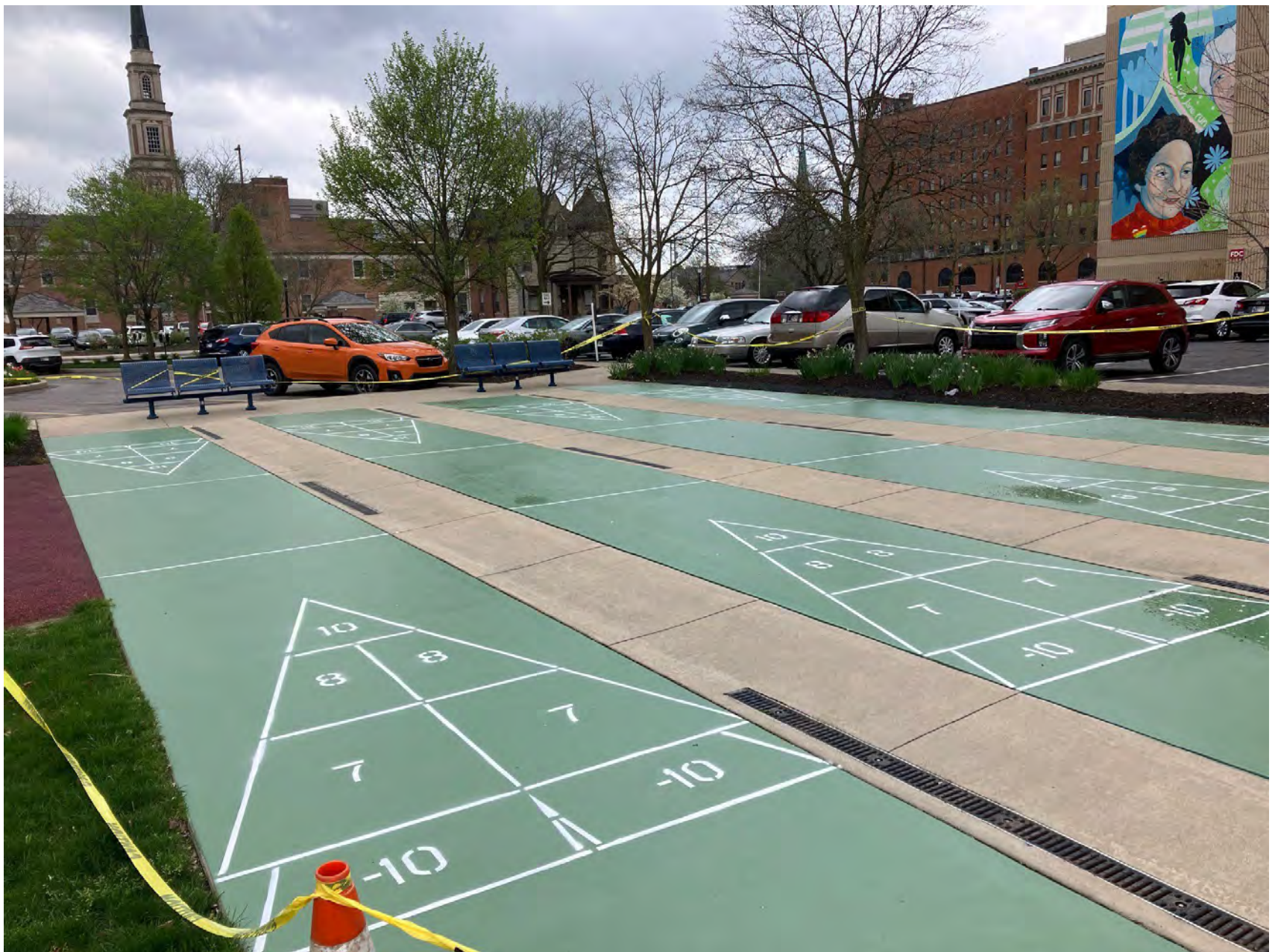
Community Center Shuffleboard Leveling & Recoating
